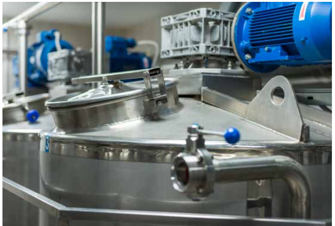
Mixing of the slurry under vacuum
